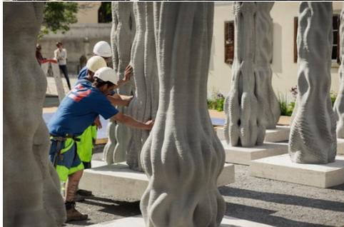
Transportation and assembly: placing the columns on-site in Riom, CH.
